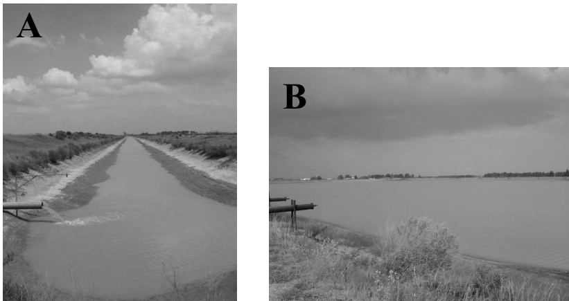
Figure 2. Tail-water recovery ditch (A) collects irrigation and rainfall runoff from fields. This water is pumped to a 15-ha reservoir (B) for future use.
